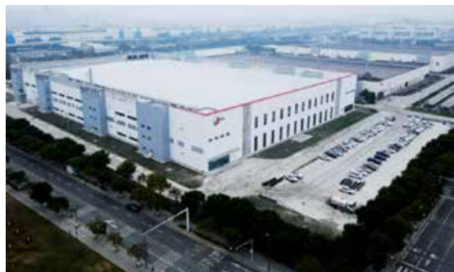
Unisem Chengdu Phase 3 construction completed
