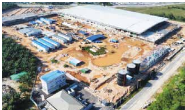
Unisem Gopeng plant construction in progress
